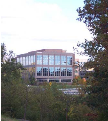
The Mass, Scale, Proportions, Color and Texture of these Buildings are Compatible with Existing Buildings Found in the MSP Historic Area.
