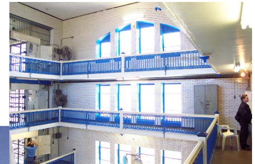
Interior View of Windows at Housing Unit 3
